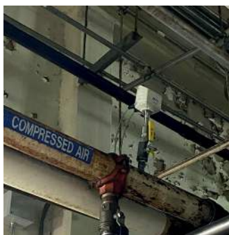
S430 Flow Meter for wet compressed air (insertion type) installation location.
